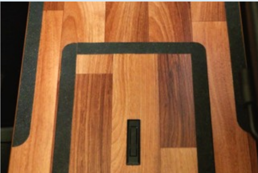
The tape is stuck onto the steps above and the floor below.
