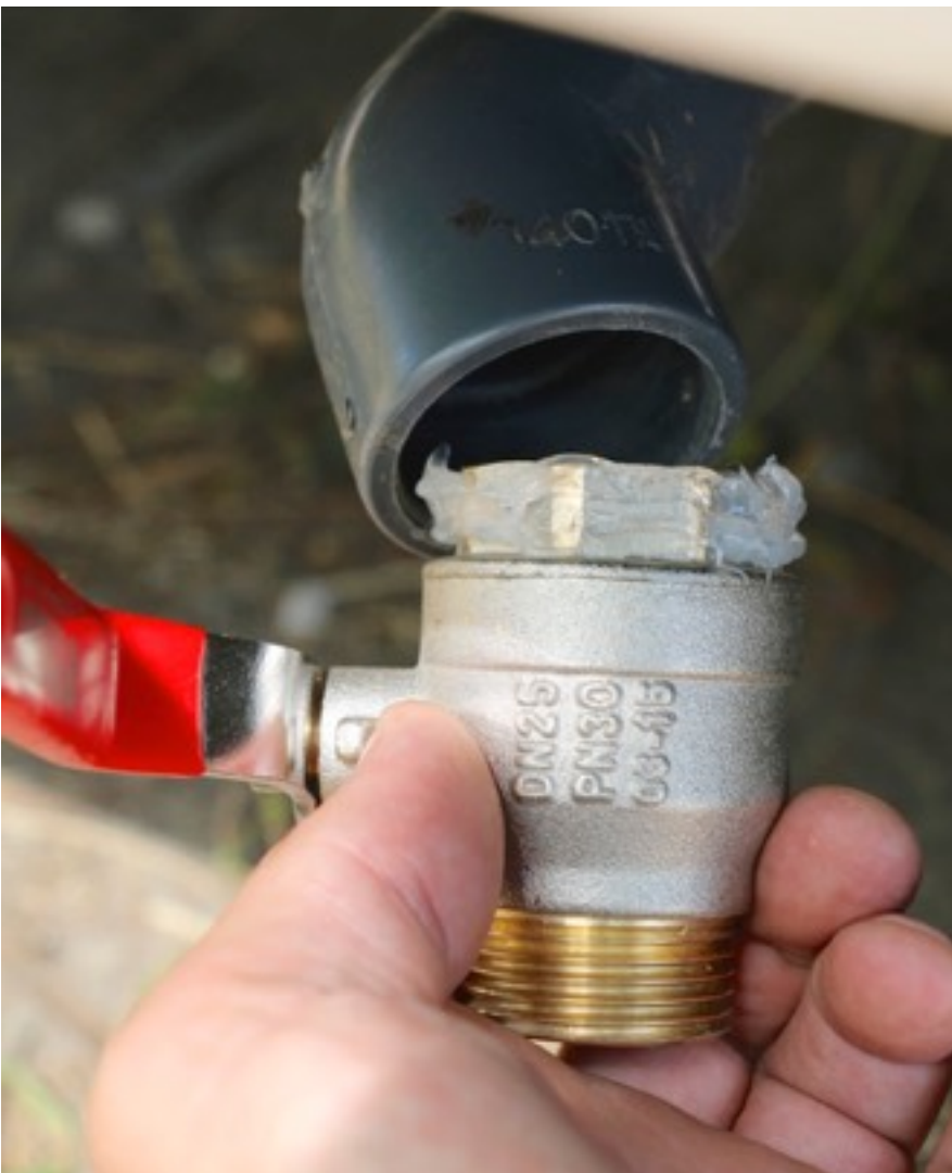
Above is existing waste pipe opening, sand this down first before assembly.
