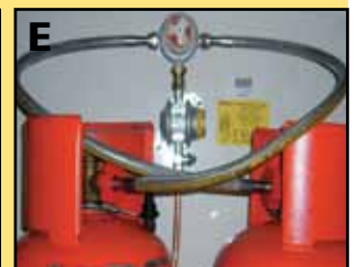
Picture shows a Truma regulator upgraded to an Auto changeover with a 01-1755 and using two propane 0.75 meter Stainless hoses. Note how the hoses cross preventing unnecessary kinking and twisting.
