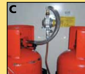
Picture shows a single 0.45m Stainless Steel hose.
