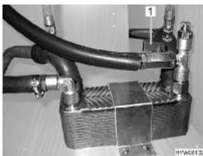
Fig. 107 Alde heat exchanger
