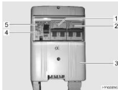
Fig. 97 240 V fuse box with safety cut-out and FI-switch
